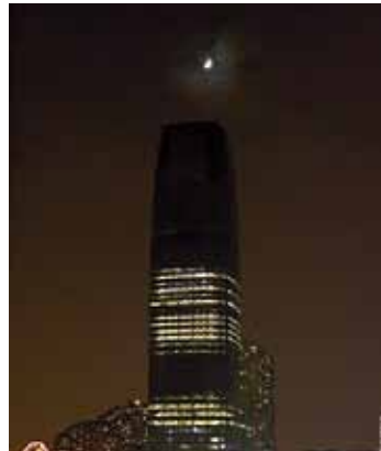
Clean buildings from the top down
