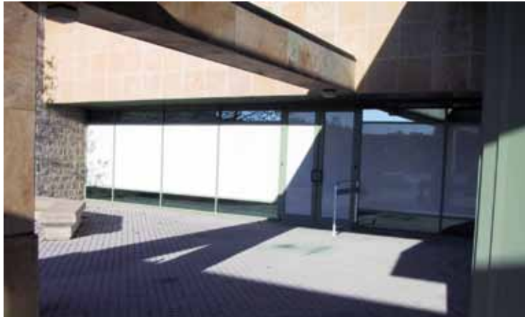
Window film eliminated collisions in this courtyard at Patuxent Refuge in Maryland
