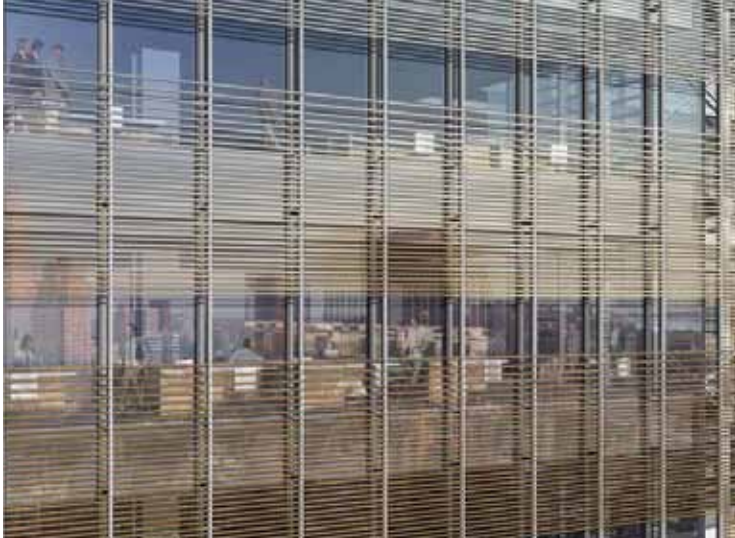
An exterior ceramic framework provides shading and daylighting (New York Times)
